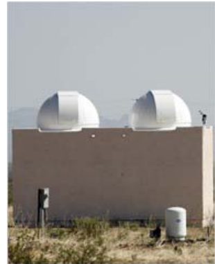
Jeff Topping for The New York Times An observatory is being built with two domes.
